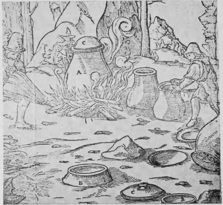
THEN — AND NOW The scene above, taken from a woodcut made in 1556, shows the smelting of oil from bitumenous rocks. Now a petroleum still is a mighty thing of steel, great heat, and high pressures, producing more in a split second than could be made in a month 400 years ago.
